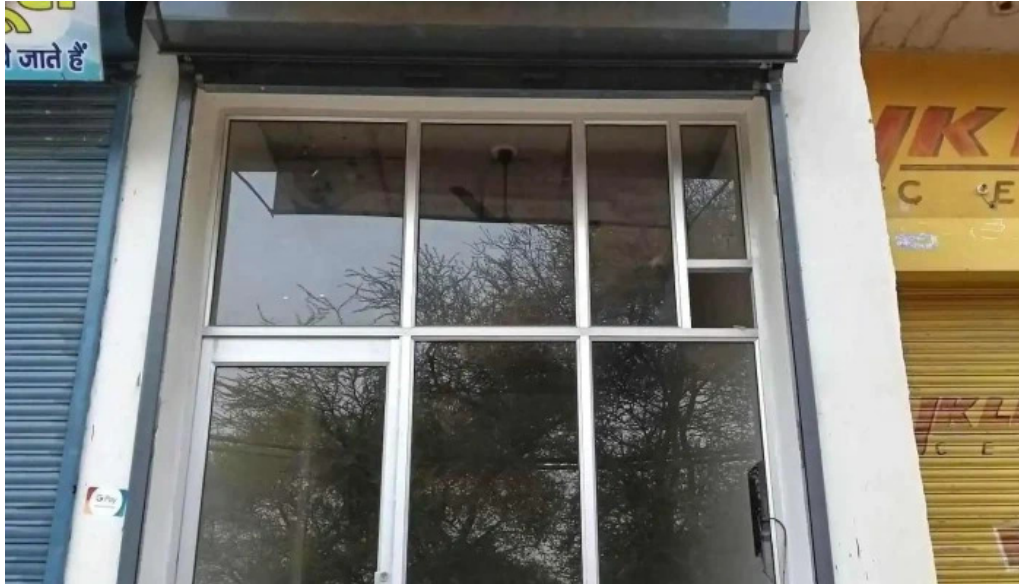
Guru laptop cctv hub all
